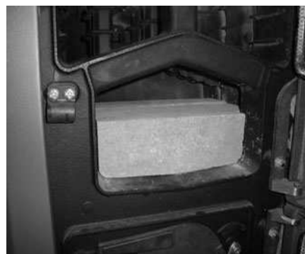
Fig. 8. Position of ceramic catalyst on the exchanger shelves in a KLIMOSZ COMBI and KLIMOSZ COMBI B boiler.
